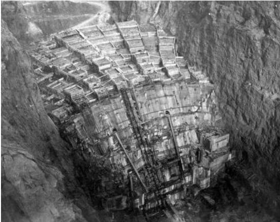
In June 6, 1933, the first round of concrete was poured for the dam's base. To allow the concrete to dry properly and prevent cracking, 230 individual blocks of concrete were poured. All in all, 3.25 million cubic yards of concrete were used, enough concrete to pave a highway 16 feet wide from New York to San Francisco.
