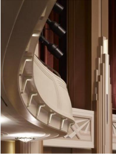
Reynolds Hall-Balcony parapet detail with stepped sidewall plaster in the background.
