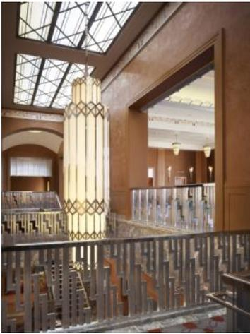
Reynolds Hall-Detail from the main stair upper landing with stainless steel framed laylight above.
