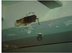
ADSW is particularly concerned about the possible effects of the planned renovations on the Ballroom. The Ballroom has not been used for many years and is in disrepair, suffering from years of neglect. At least two areas of serious decay are clearly visible in the ceiling. Specific issues related to the Ballroom include:
